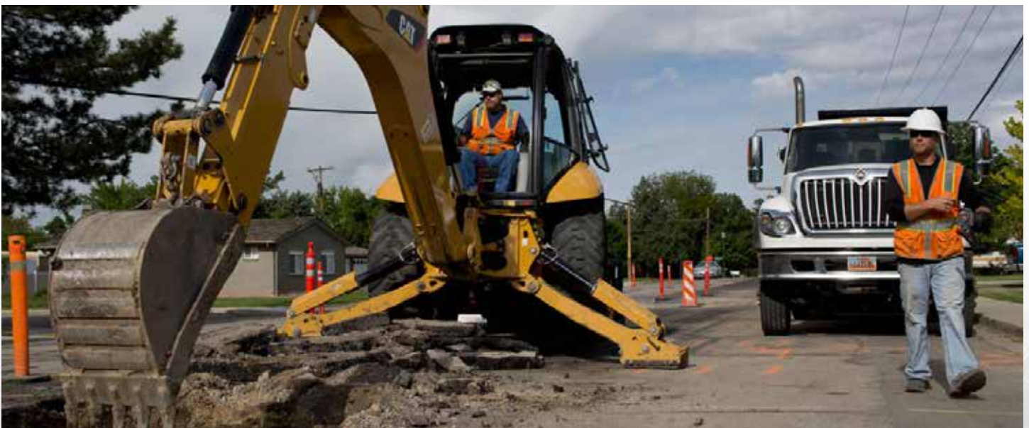
Orem Public Works Crew Members Help Install a New Water Line
